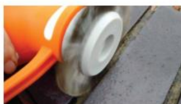
Masonry Grout Cleaning
